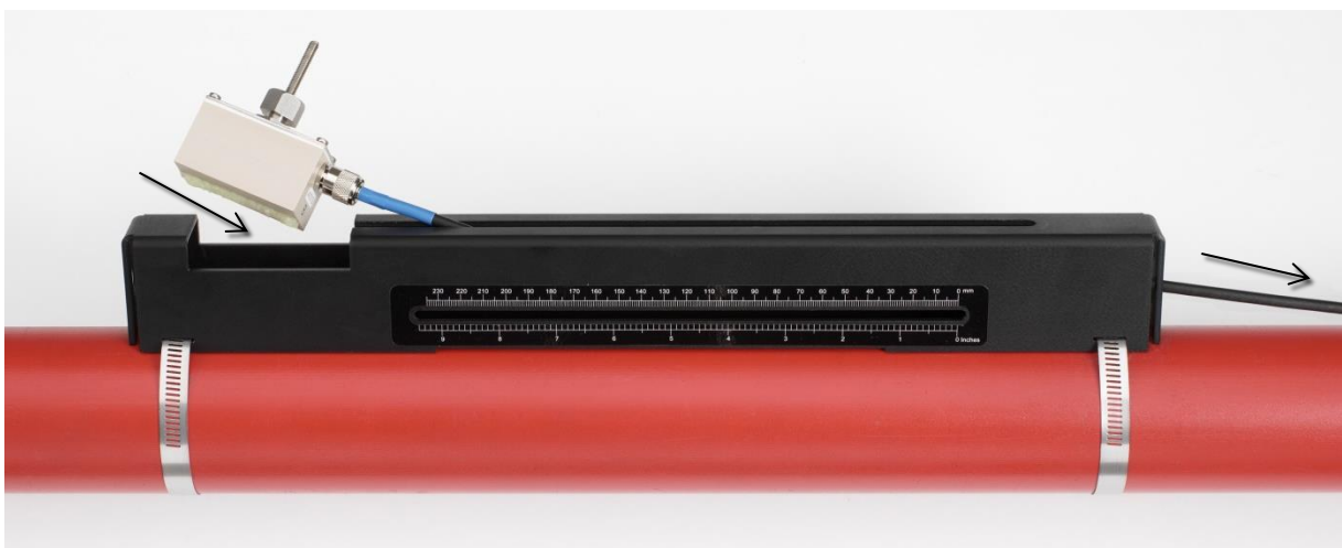
Figure 13 Installing downstream (blue) transducer
