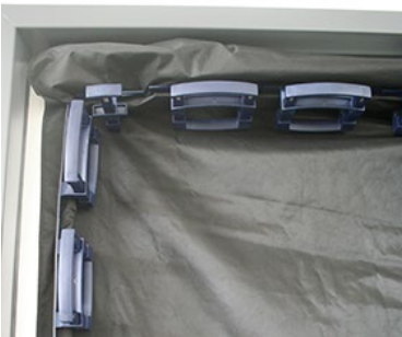
Fig. 18: Wide and narrow clamps positioned
