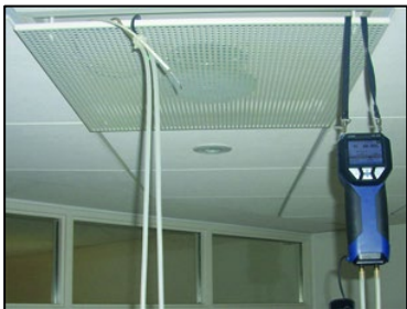
Fig. 33: Example - Fixing with the supporting loop
