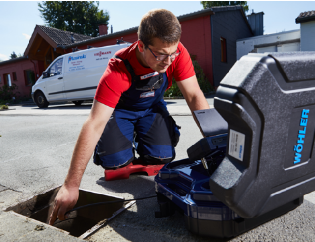
Secure drain inspection with the waterproof camera head.
